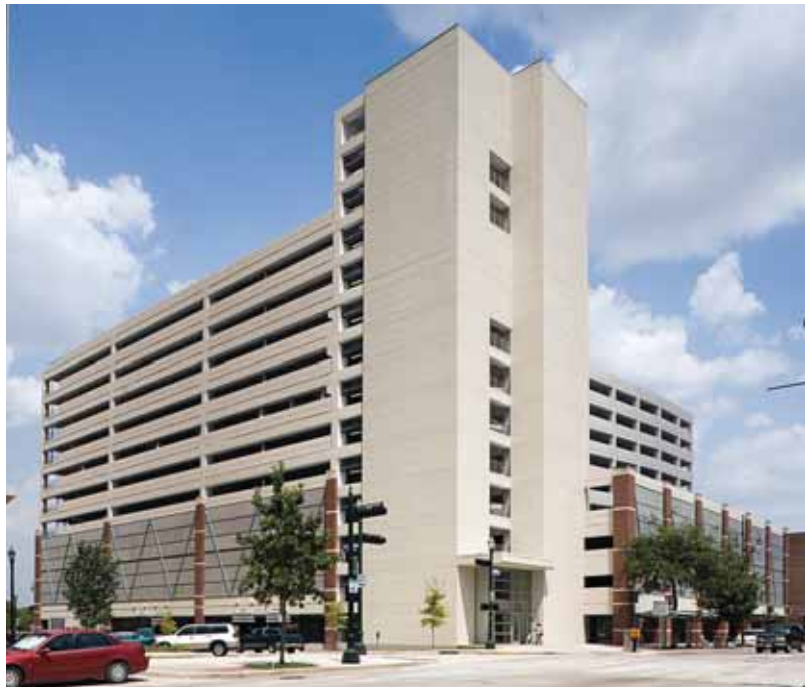
Adding to the garage's aesthetic appeal are the reveals in the cast-in-place concrete bumper walls used to avoid the "monolithic" look of 12 levels of concrete. © Richard Payne
