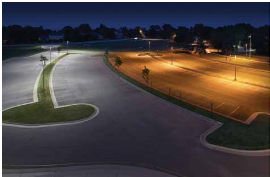
LED lighted area (L) and HID side by side.
