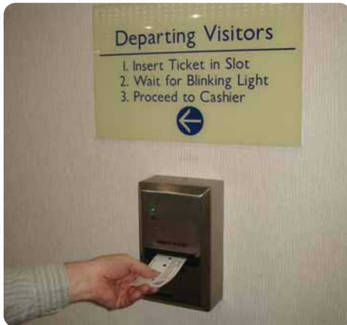
Parkers dip their tickets when they leave the elevator lobby – This puts the number on the display above and prompts attendants to bring the car around.
