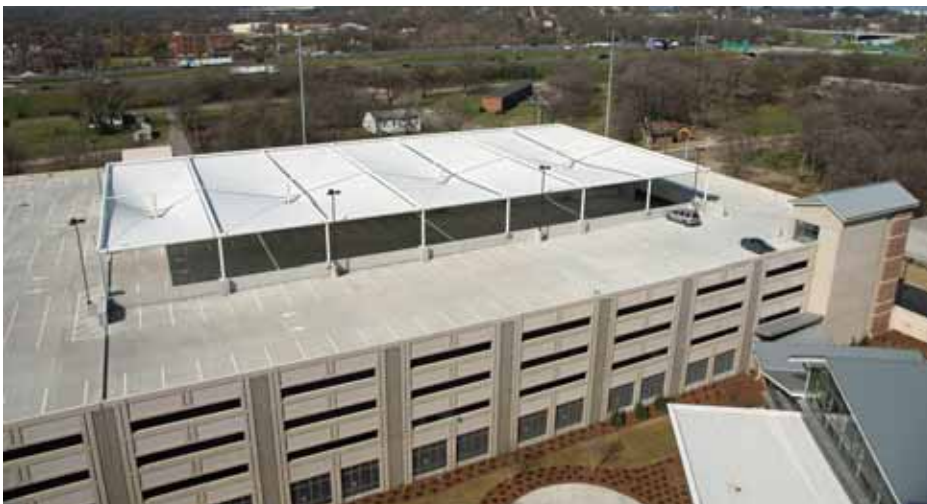
The Social Security Administration parking structure in Birmingham, AL, features a sustainable design using a total precast concrete structure that will help it obtain LEED certification. It includes a rooftop rainwater-collection system used for irrigating a rooftop garden on a new low-rise office building nearby. The 456,618-square-foot project was designed by HOK Architects and OPUS Architects & Engineers. Photo courtesy of Metromont Corp.
