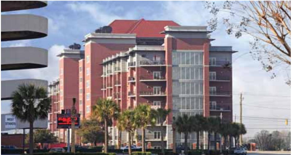
The Carolina Walk condominium project on the University of South Carolina campus in Columbia features a total precast concrete building system to create multifamily housing and parking facilities. The project, designed by Ard, Wood, Holcombe & Slate Architects, features precast concrete panels that combine contrasting architectural finishes using sandblasting and brick form liners with field-applied stain. Photo courtesy of Metromont Corp.
