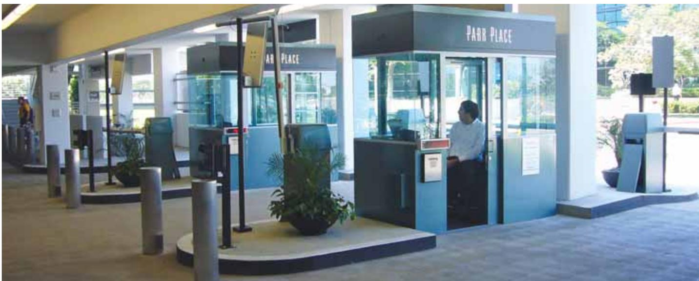
Typical design for a medium-size facility, one dedicated in lane, one dedicated out lane and one reversible lane in the middle. Pay-on-exit doesn't mean that the system isn't high-tech. Note the antennae for automatic vehicle identification (AVI).
